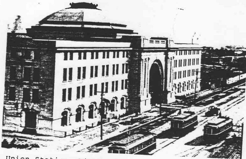
4 Union Station, Winnipeg, front elevation, ca. 1911. (National Archives of Canada - hereafter NA - PA21730.)
